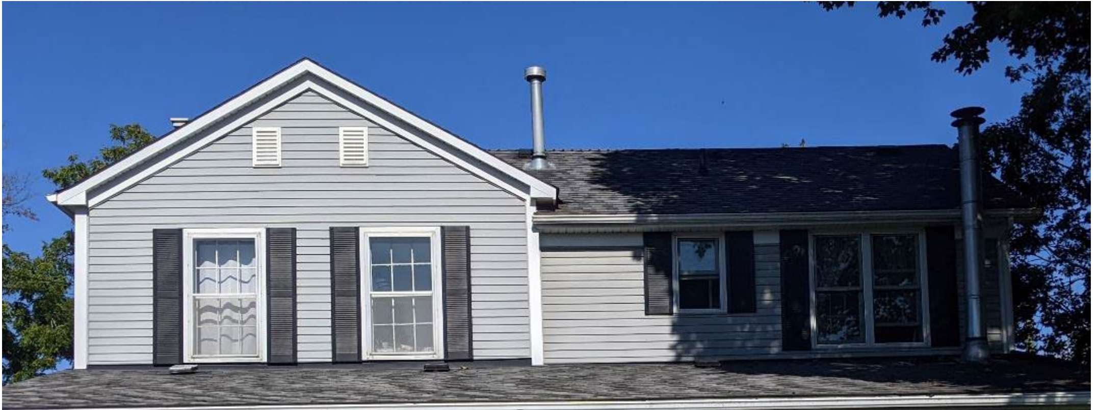
Windows at Rear Elevation
