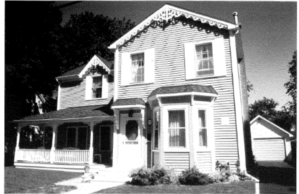
This Victorian Style home was built in two stages. The original building, right, has a side hall entrance with a one-storey window. Note the decorative brackets at the entrance canopy and the bay window – also the decorative scrollwork on the front gables. The addition, or ell, at left was built more recently.
