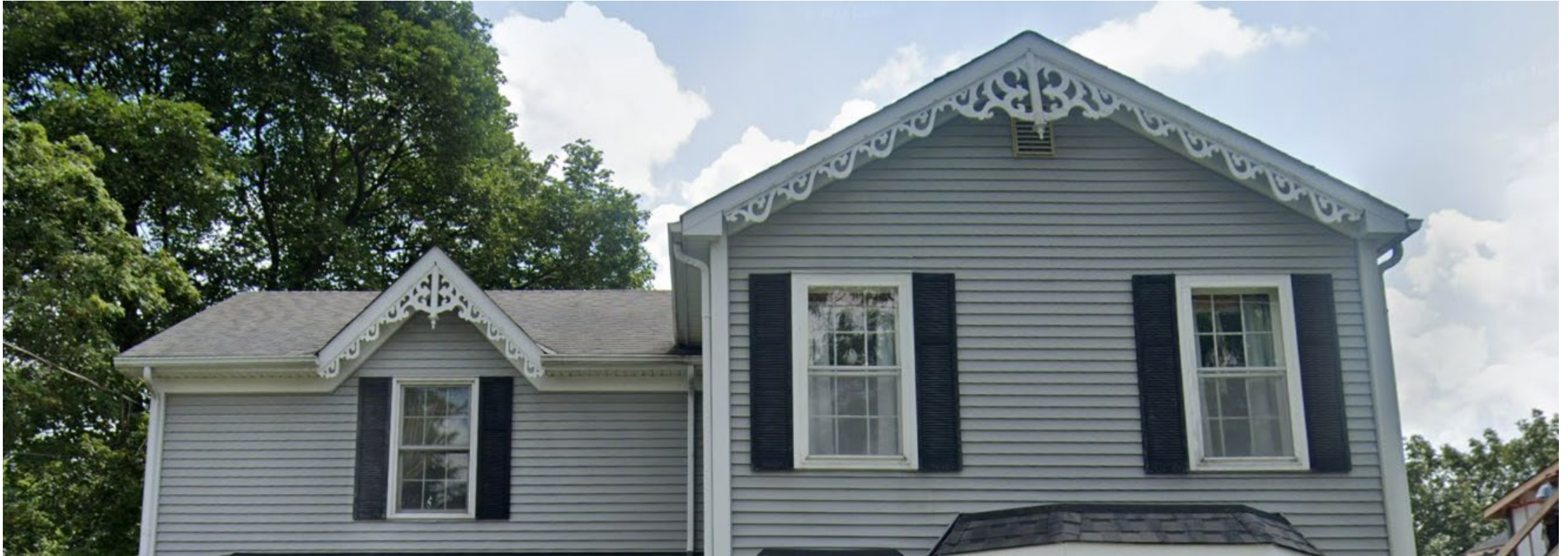
Windows at Front Elevation
