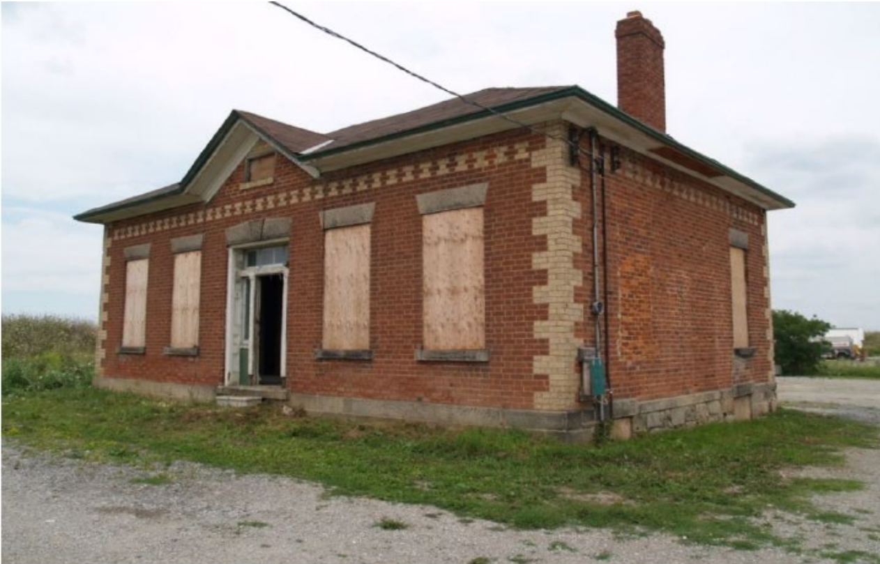
West and South Façade Before Rehabilitation
