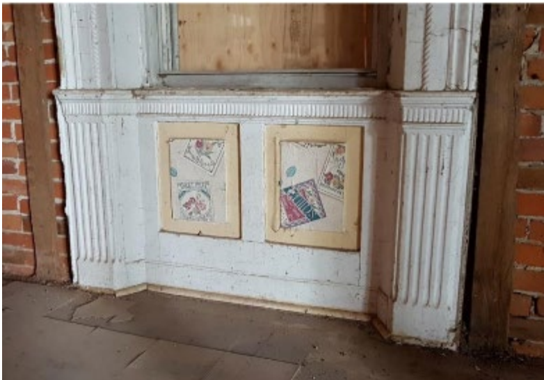
Prior to restoration
