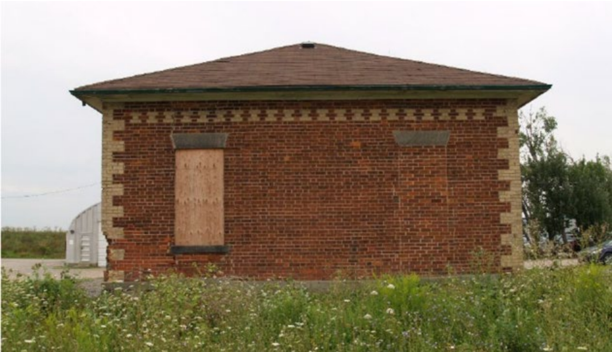
North Façade Before Rehabilitation
