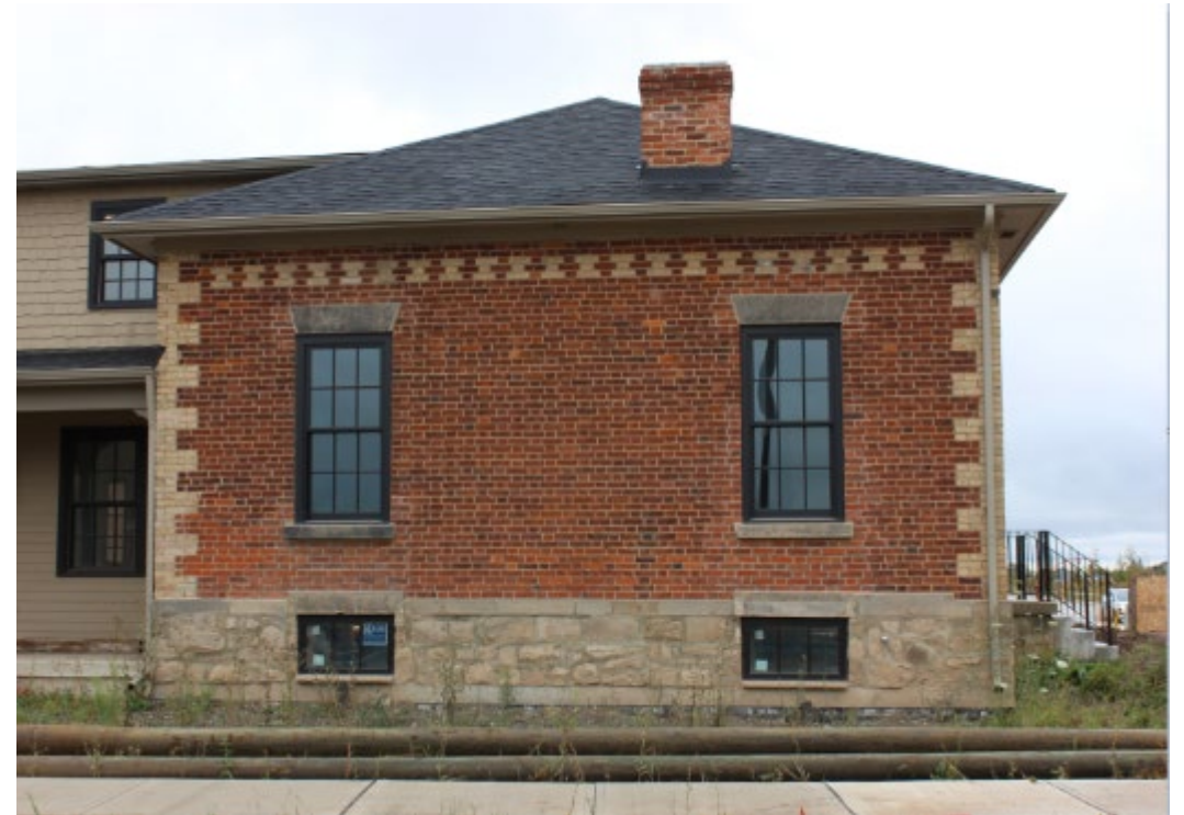
North Façade After Rehabilitation
