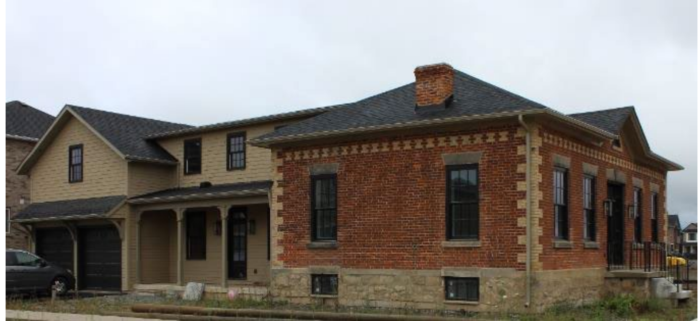
North East Façade After Rehabilitation
