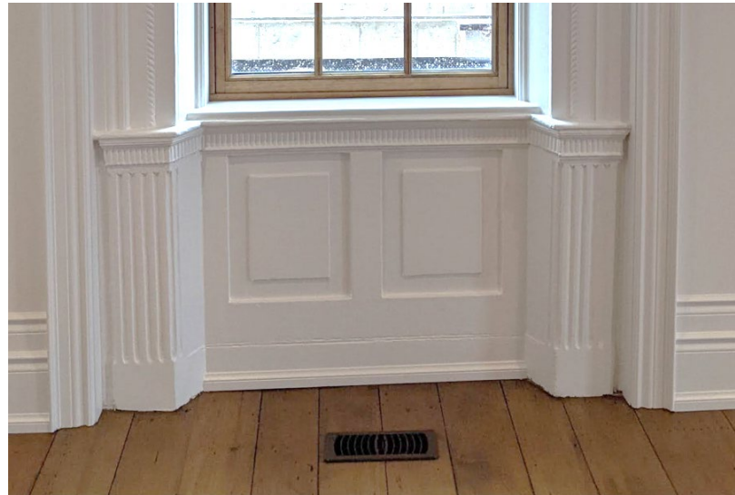
Restored Window Casing
