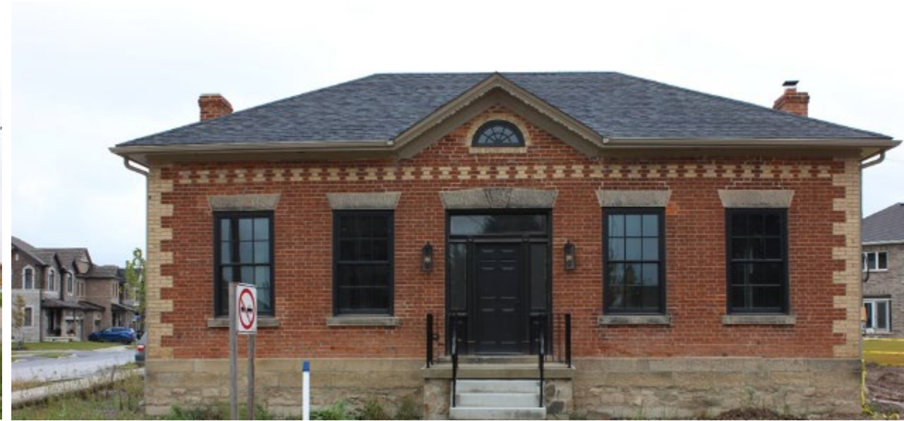
West Façade After Rehabilitation
