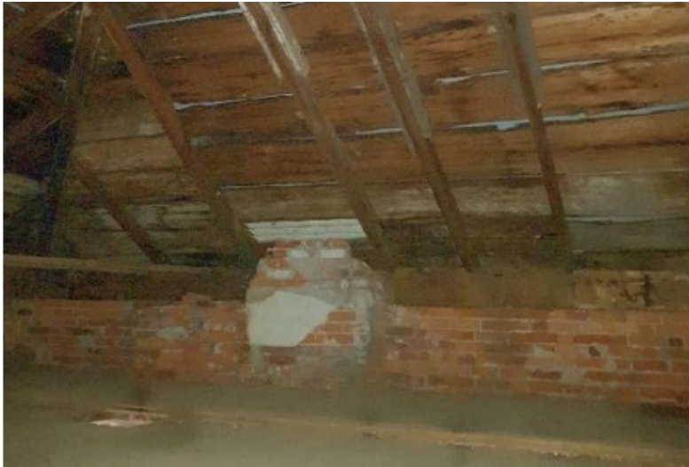
Condition of Attic prior to rehabilitation
