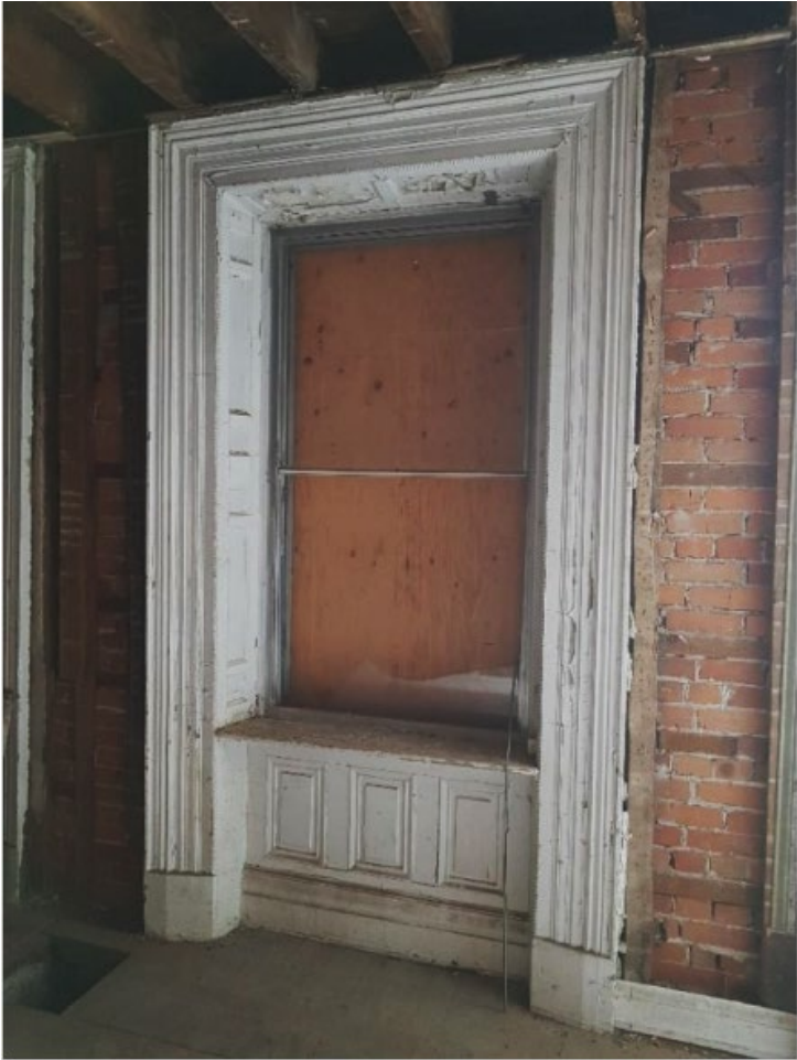
Prior to restoration
