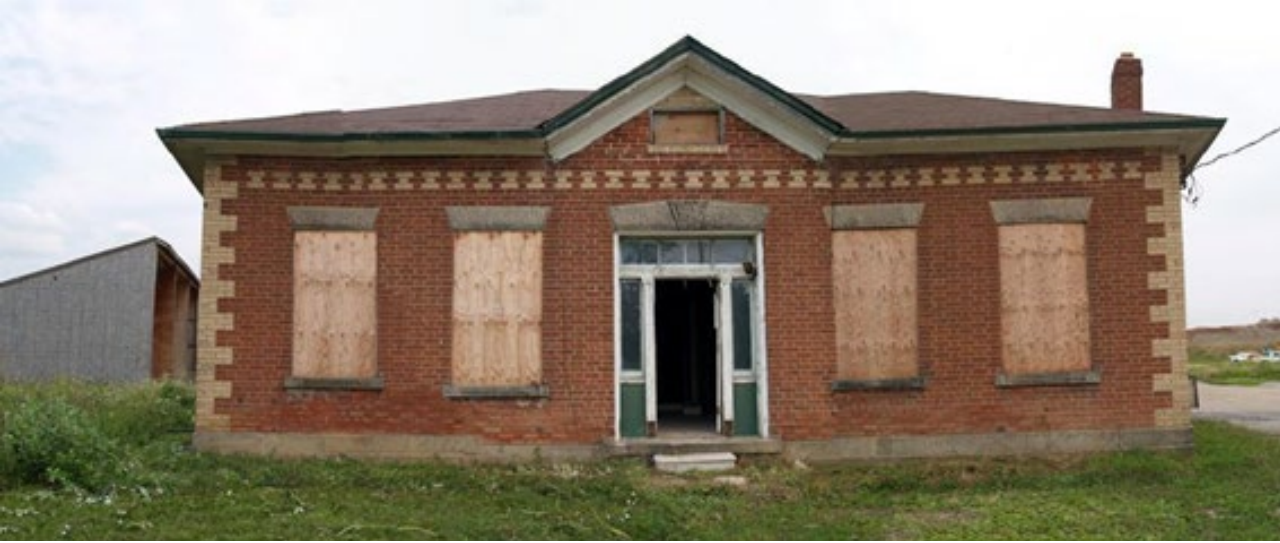
West Before Rehabilitation
