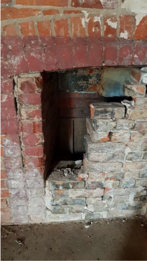
Prior to restoration Fireplace 1
