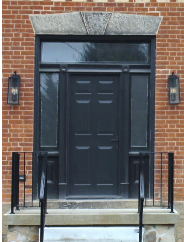
Restored Front Door Exterior
