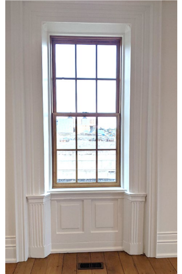
Restored Window Casing
