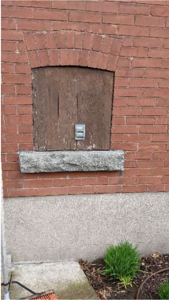
Window at West elevation
