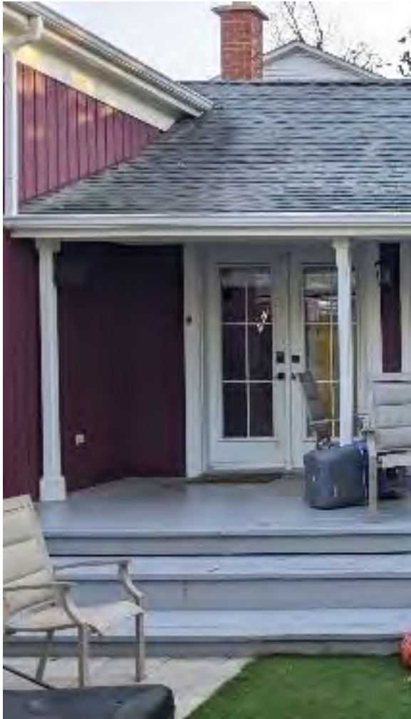
Brick Chimney view from interior courtyard
