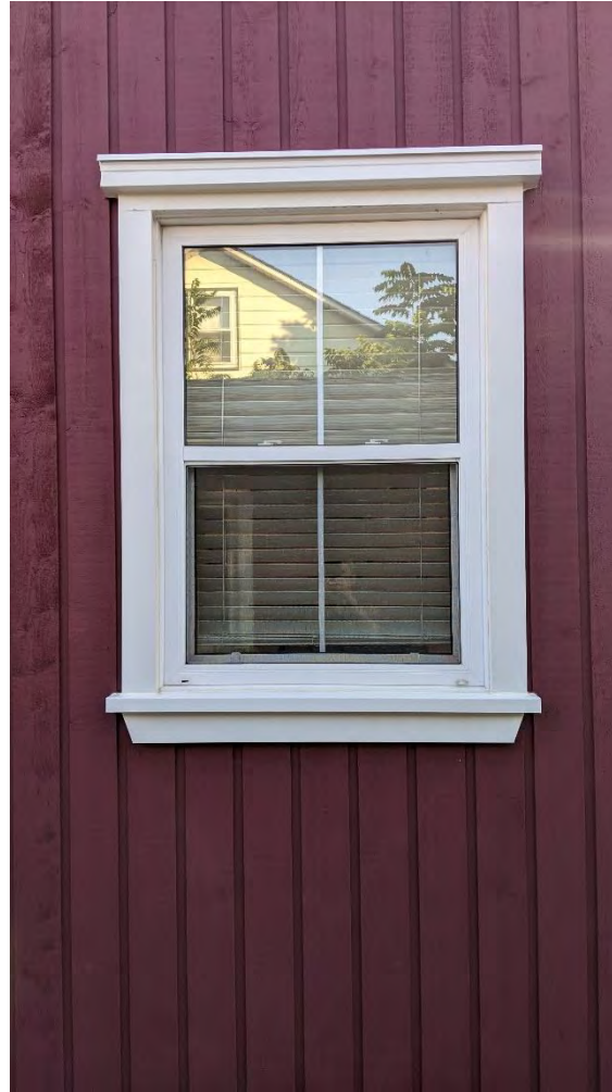
East elevation Window Ground
