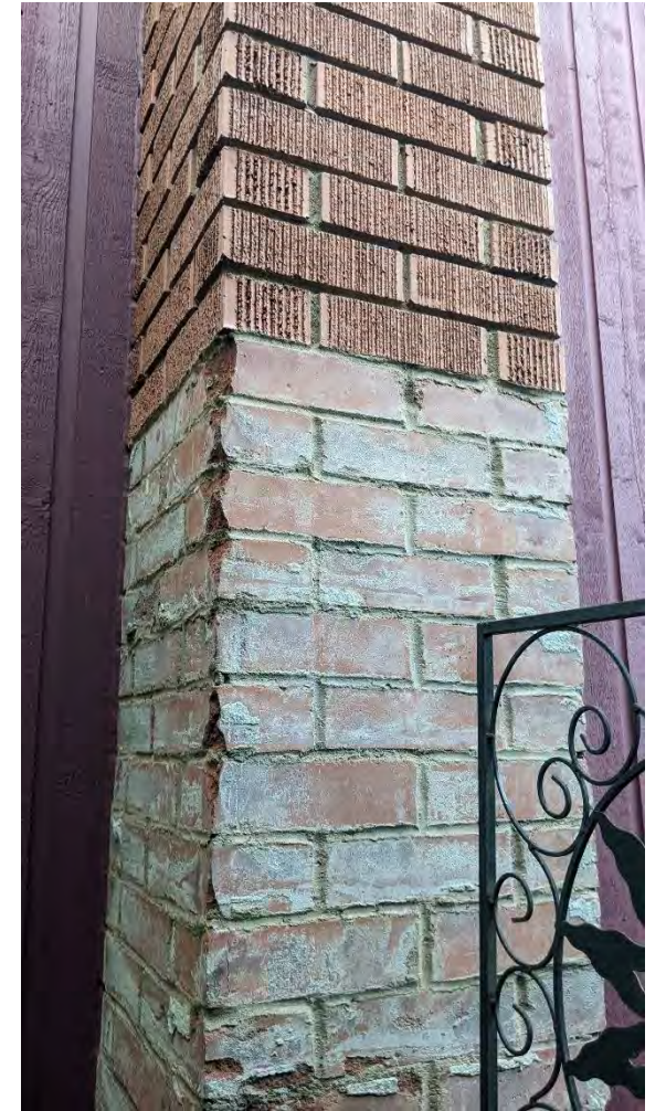
Brick Chimney Base
