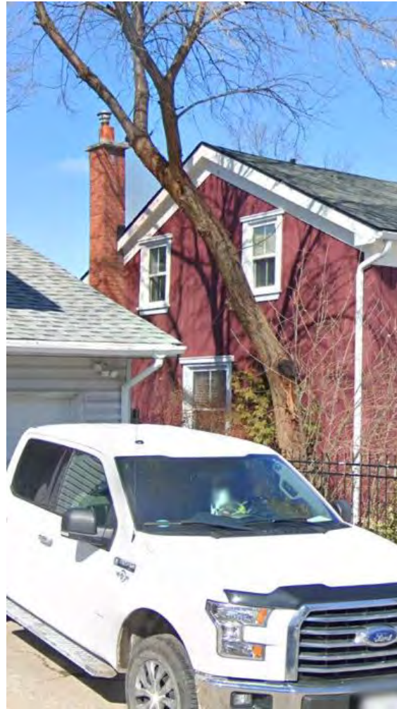
Brick Chimney at West Elevation
