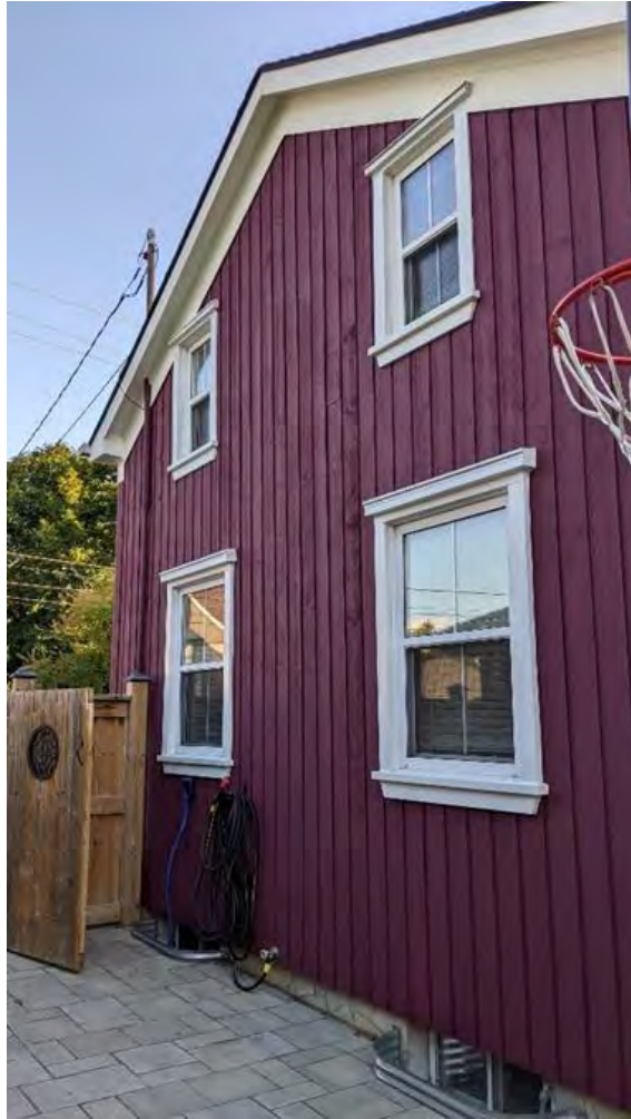
South Elevation Window
