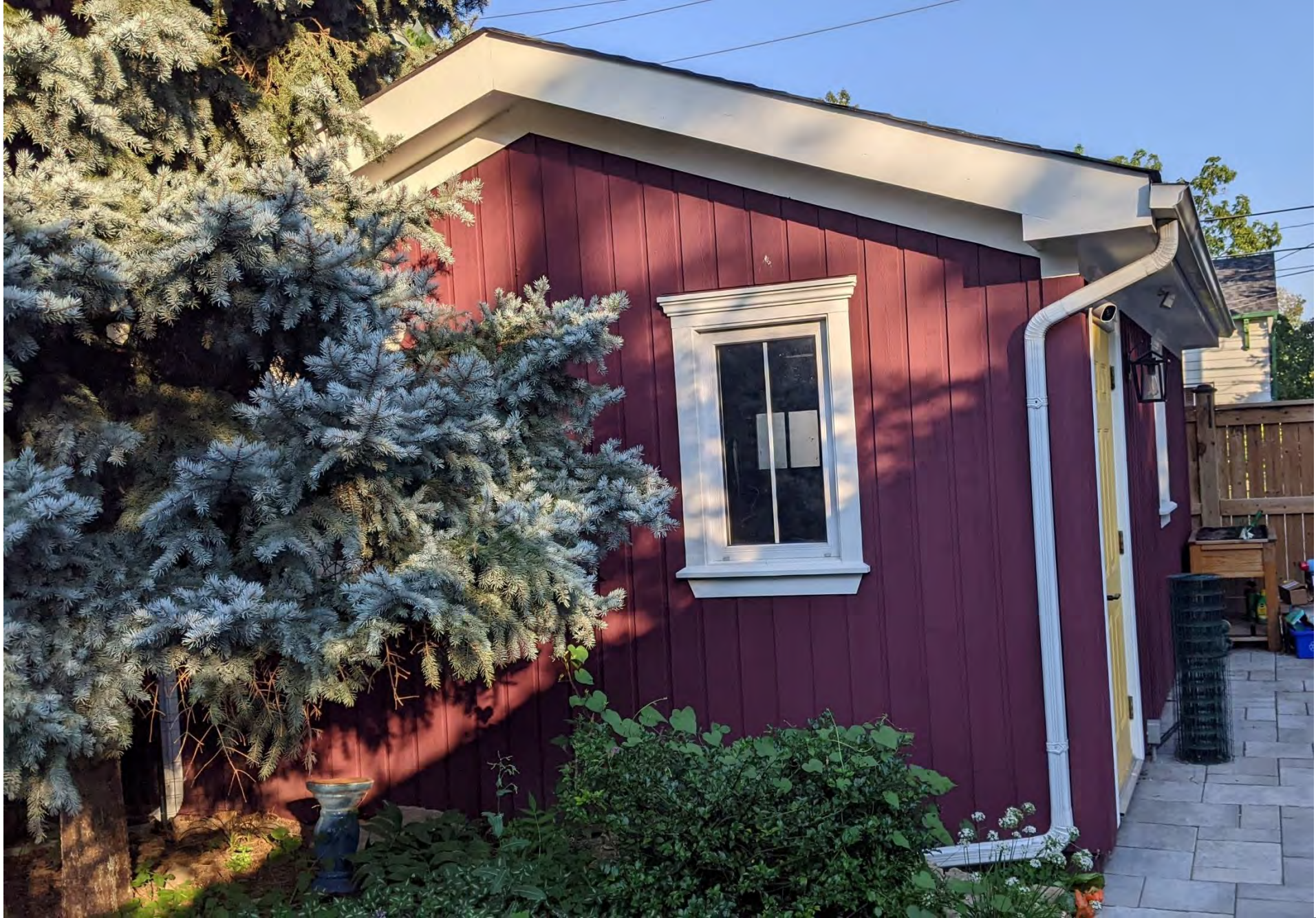
Existing Garage Non Heritage View from Interior Courtyard
