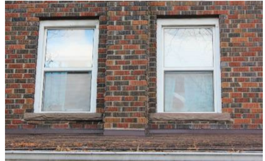
Rear Windows Upper Floor
