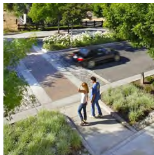
Barrier Free curb ramps and crossing, and at-grade barrier-free building entrance help to make a place more accessible to all users
