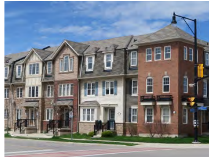
Townhouses and live-work type buildings should be strategically interspersed throughout Evolving Neighbourhoods and employed at key locations such as around village squares and along collector roads
