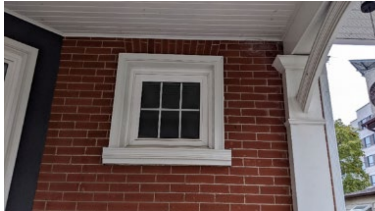
Window details at Front Porch
