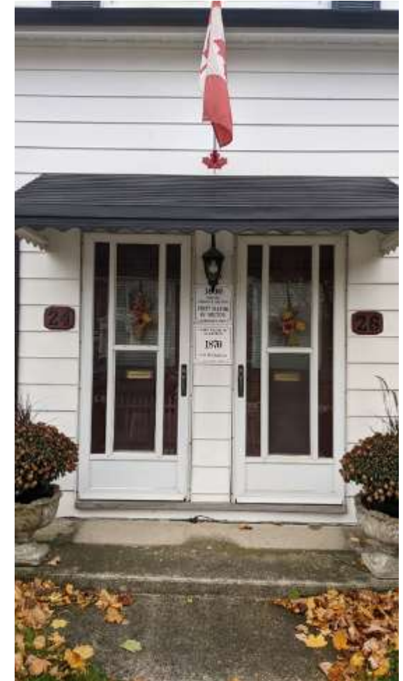
Two Entrance Door
