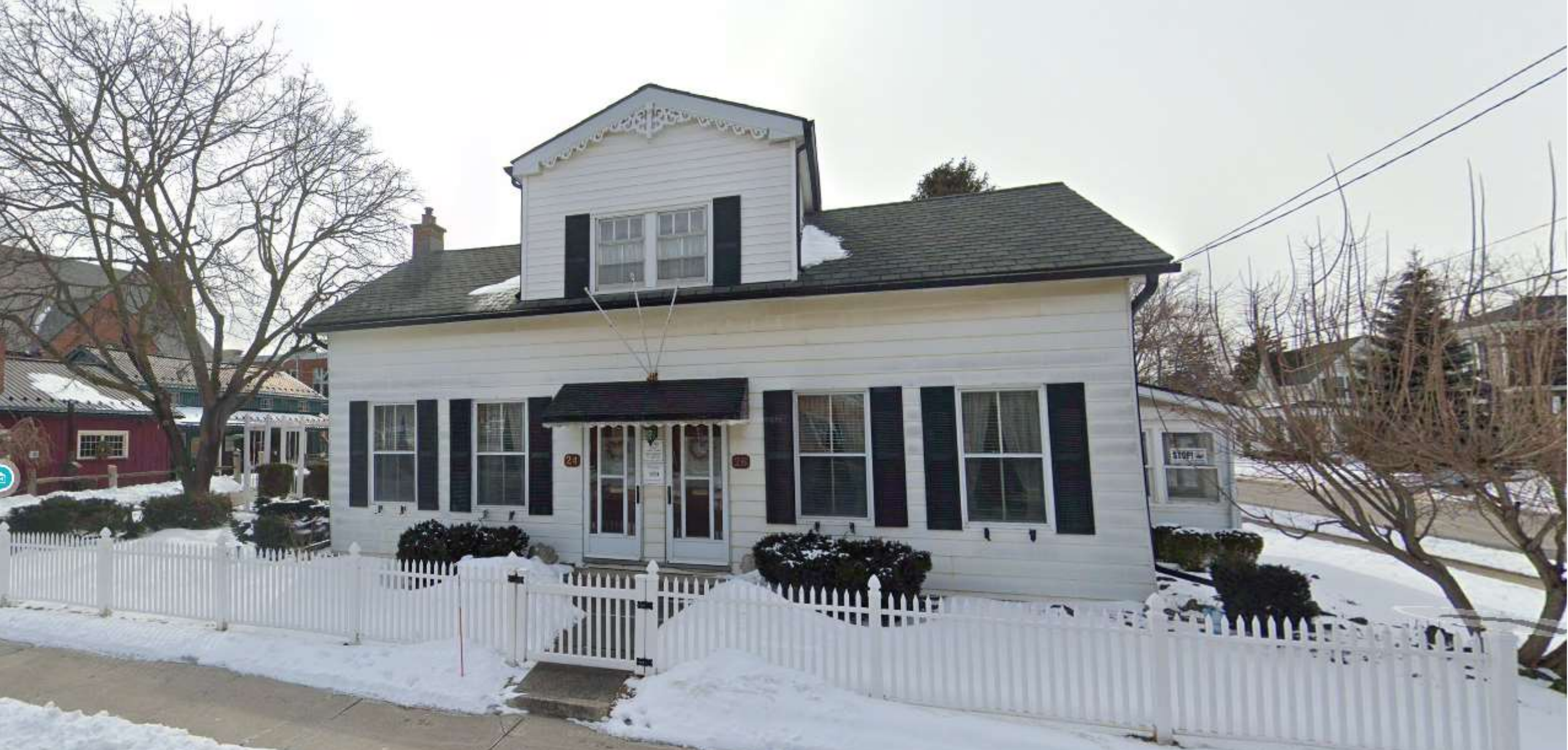
Appendix 3 Photographic Record _ Heritage Attributes _ 24 and 26 James Street
