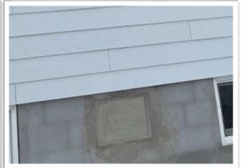
Location of Builder's engraving on North Elevation
