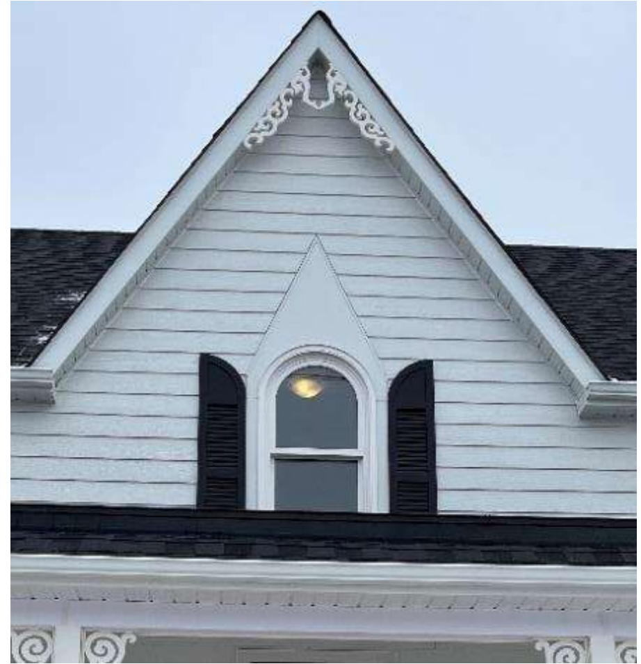
North East Façade After Rehabilitation
