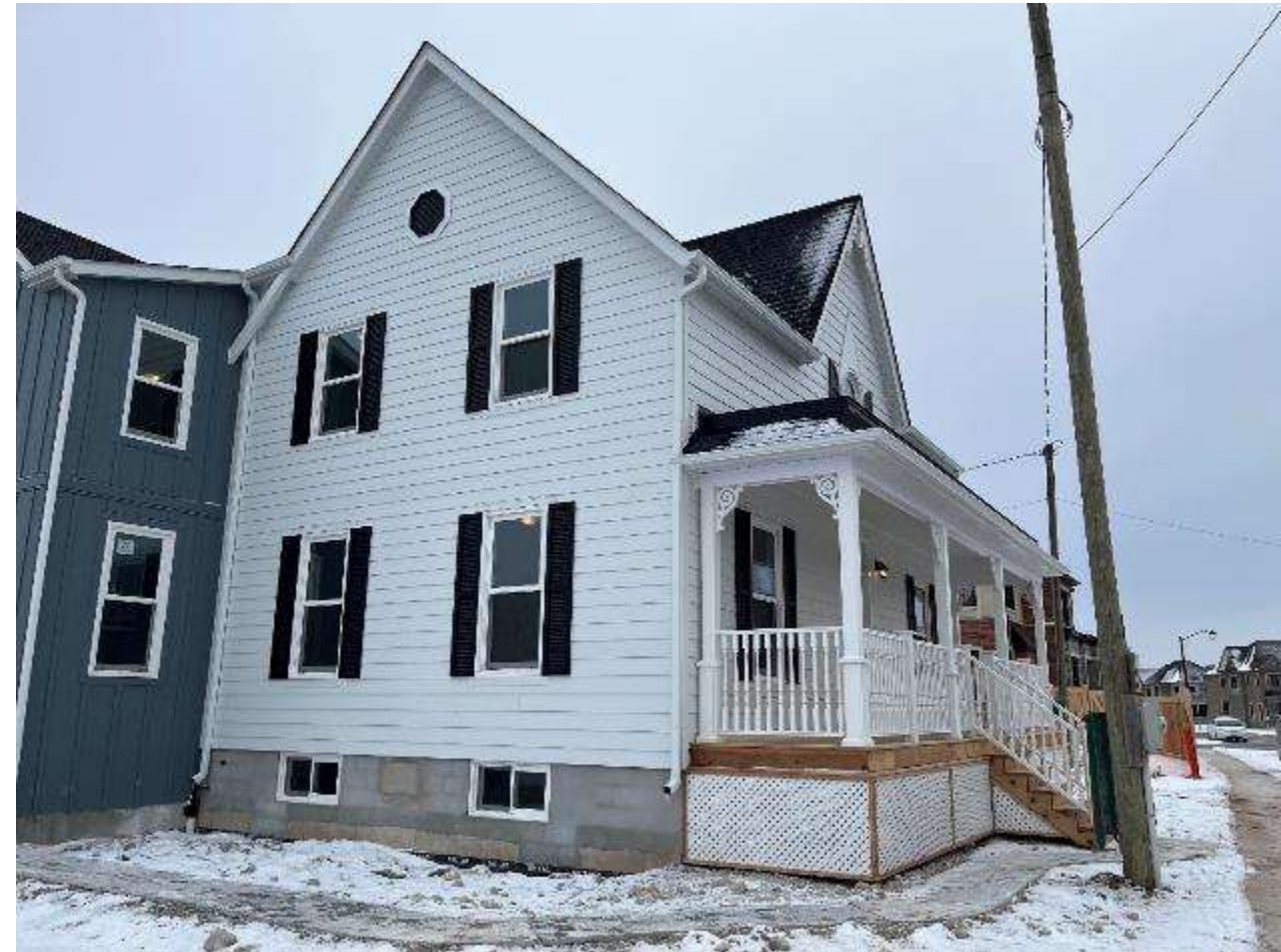
North Façade After Rehabilitation
