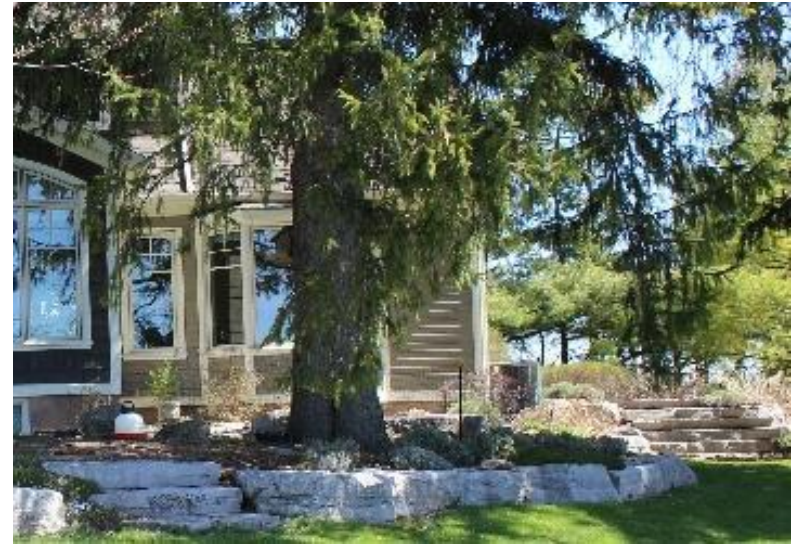
South West Elevation (Rear Addition)
