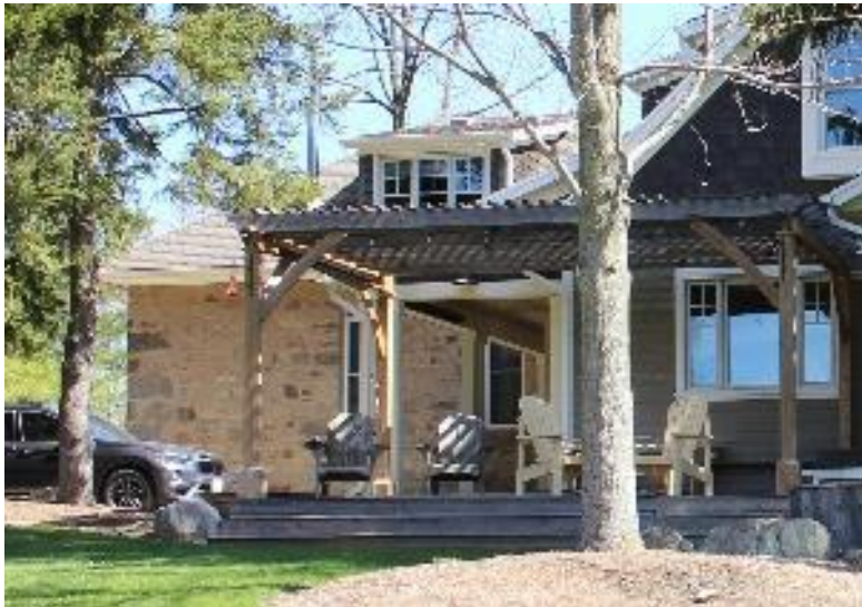
South West Elevation (Rear Addition)
