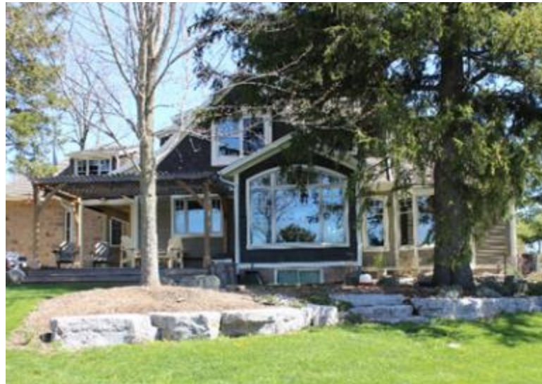
South West Elevation (Rear Addition)
