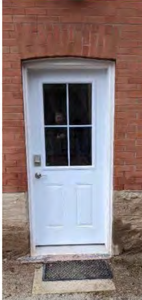
New Door with arch brick header
