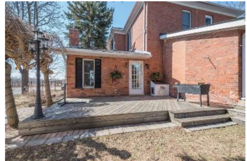
Rear View showing additions
