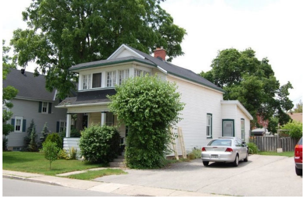
The original form, rooflines and massing of the one and a half storey house exterior
