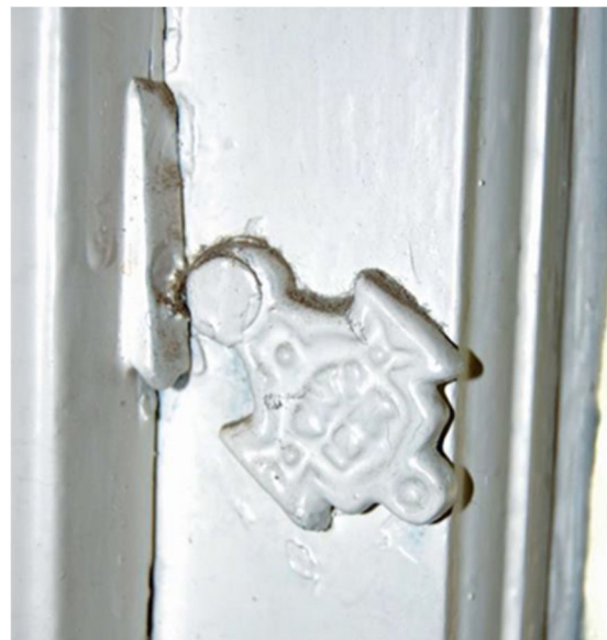
Window sash locks with patent date of "1874"
