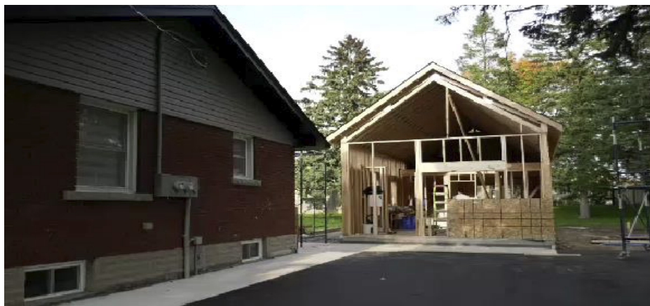
Figure 4: A tiny home under construction in the City of Kitchener
