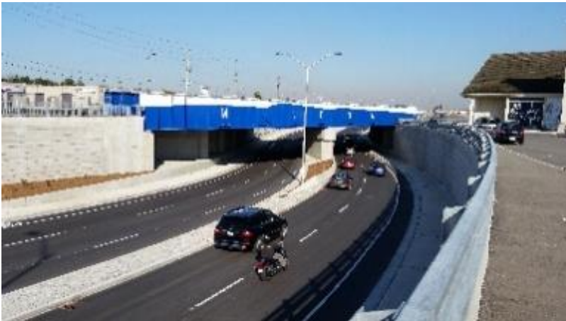
Figure 2. Cars driving under Milton bridge.
