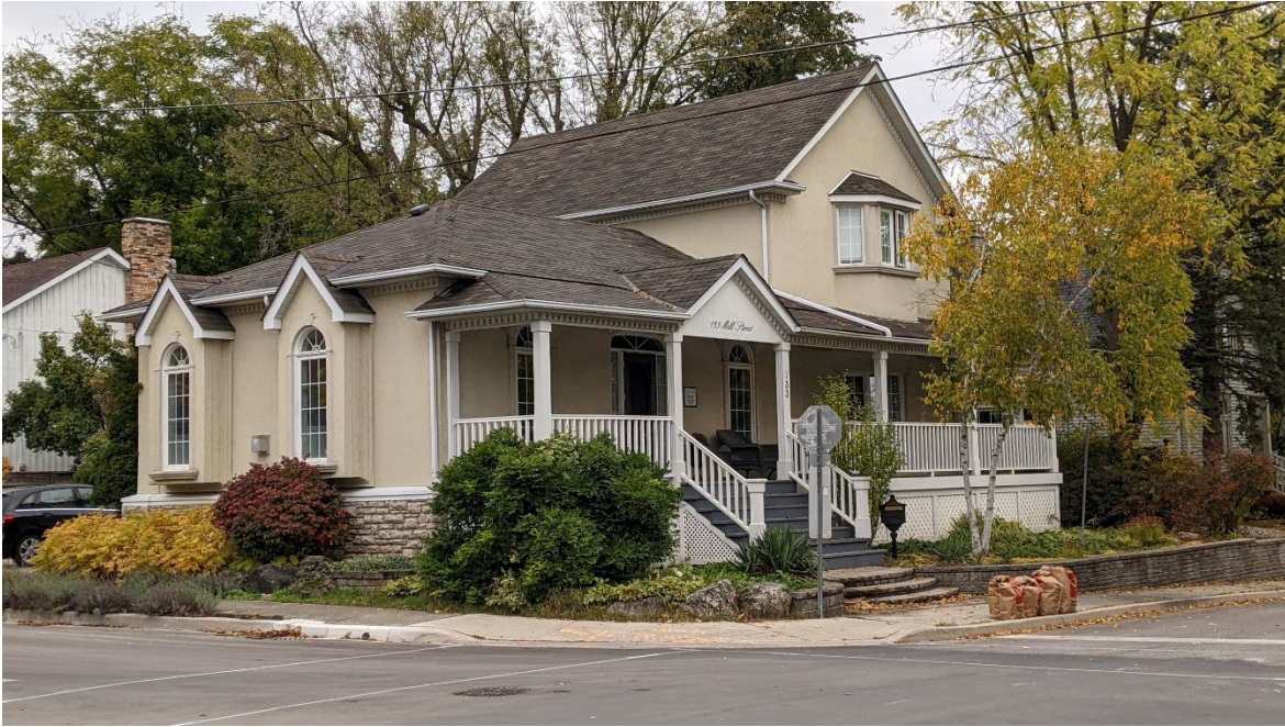
Figure 1 View of 133 Mill at the corner of Mill and James Street
