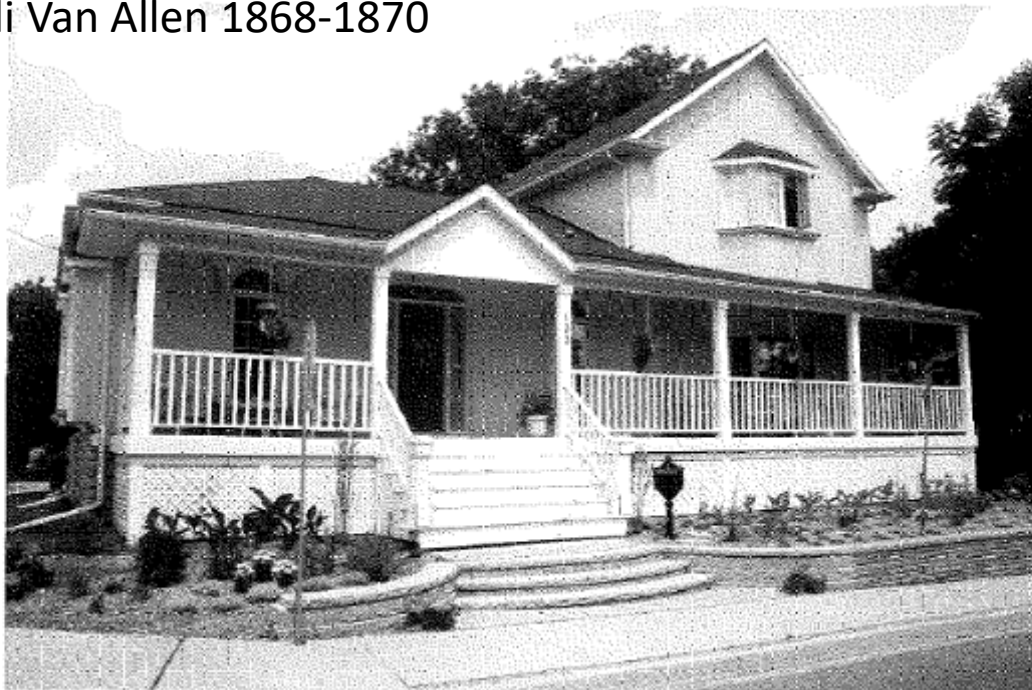
An original Regency cottage on a high base has disappeared in recent major additions. The original section of the building was to the left of the photo.
