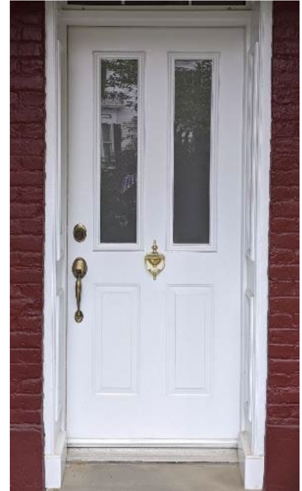
Single Leaf Four Panels Door with glass inserts
