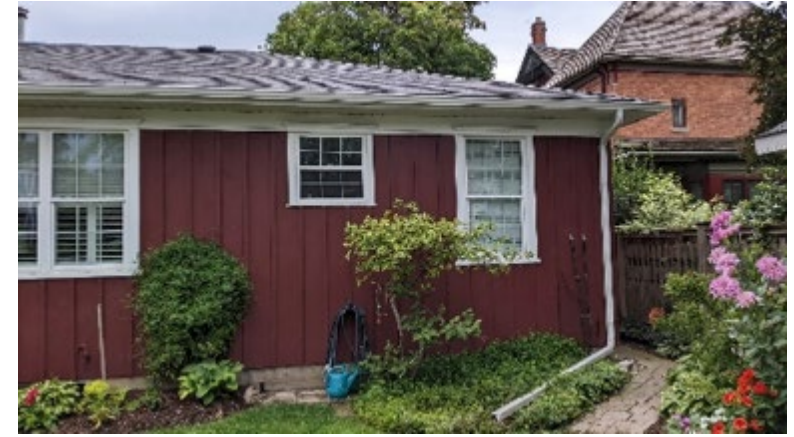
South Elevation (1995 additions)
