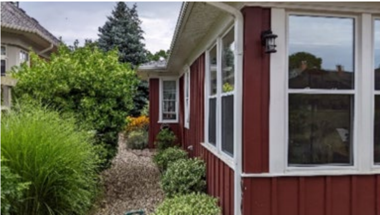
West Elevation (1995 additions)
