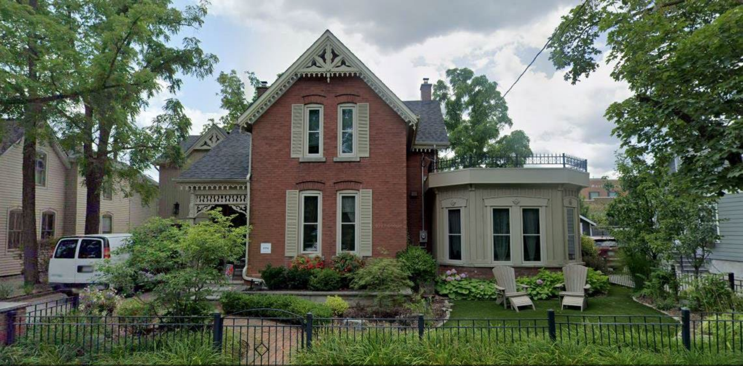
Appendix 3 Photographic Record _ Heritage Attributes _ 168 Martin Street
