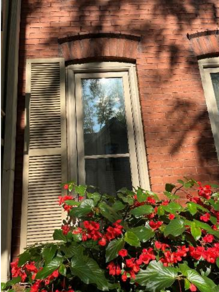
Ground Floor Left Flank Window
