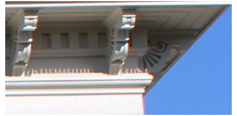
Decorated roof brackets _ Right Corner
