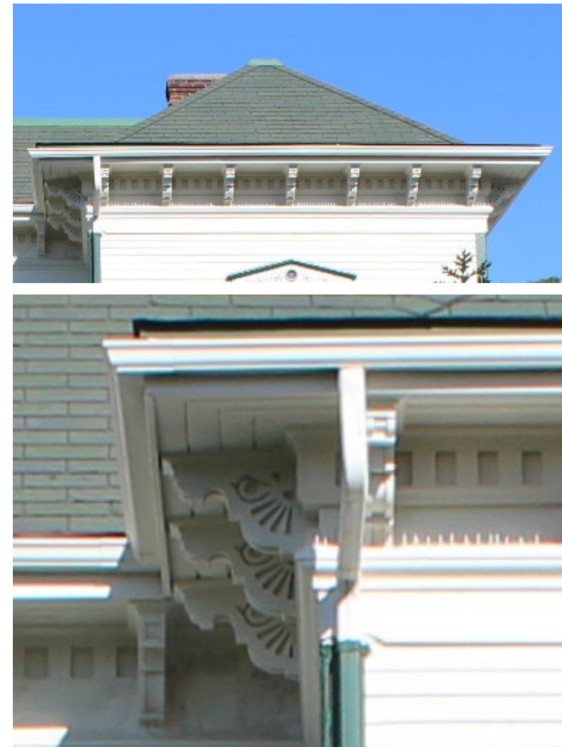
Hip roof with decorative eaves bracket
