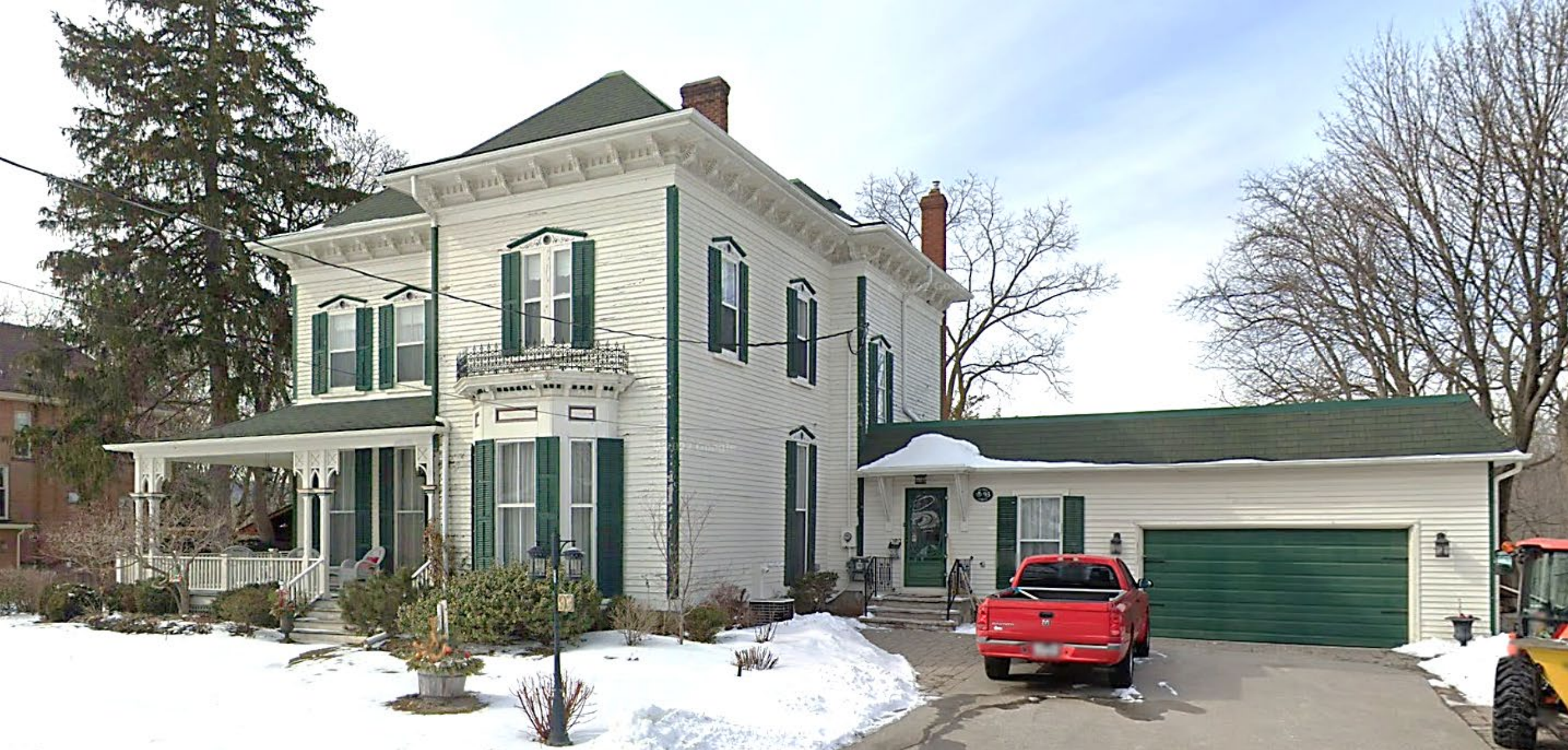
Appendix 3 Photographic Record _ Heritage Attributes _ 93 Victoria Street
