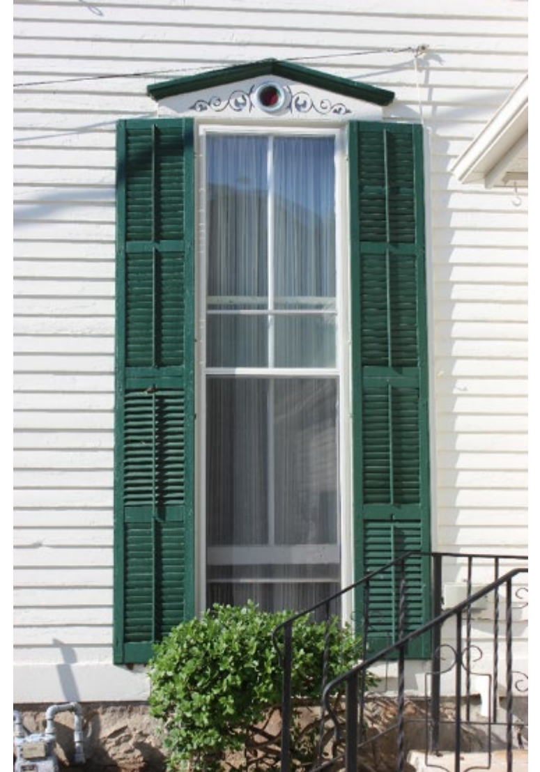
Ground Floor East Elevation Window
