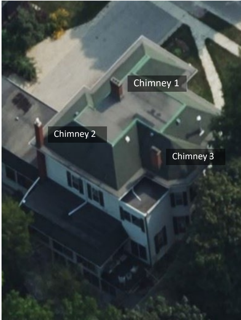
Location of Chimneys
