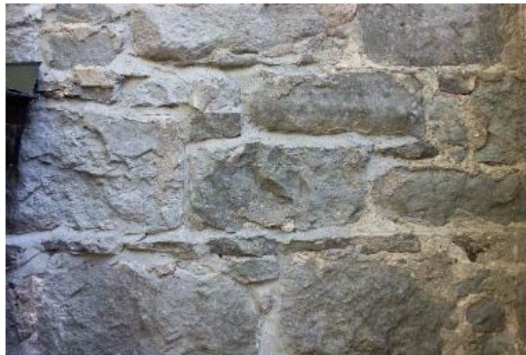
Exterior random rubble stone wall
