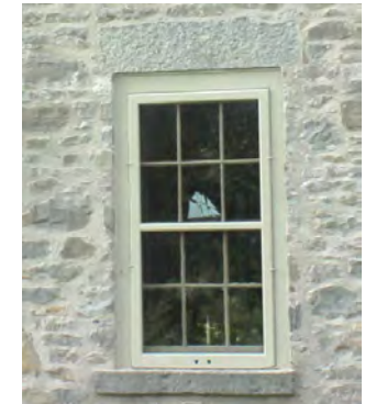
East Elevation Windows
