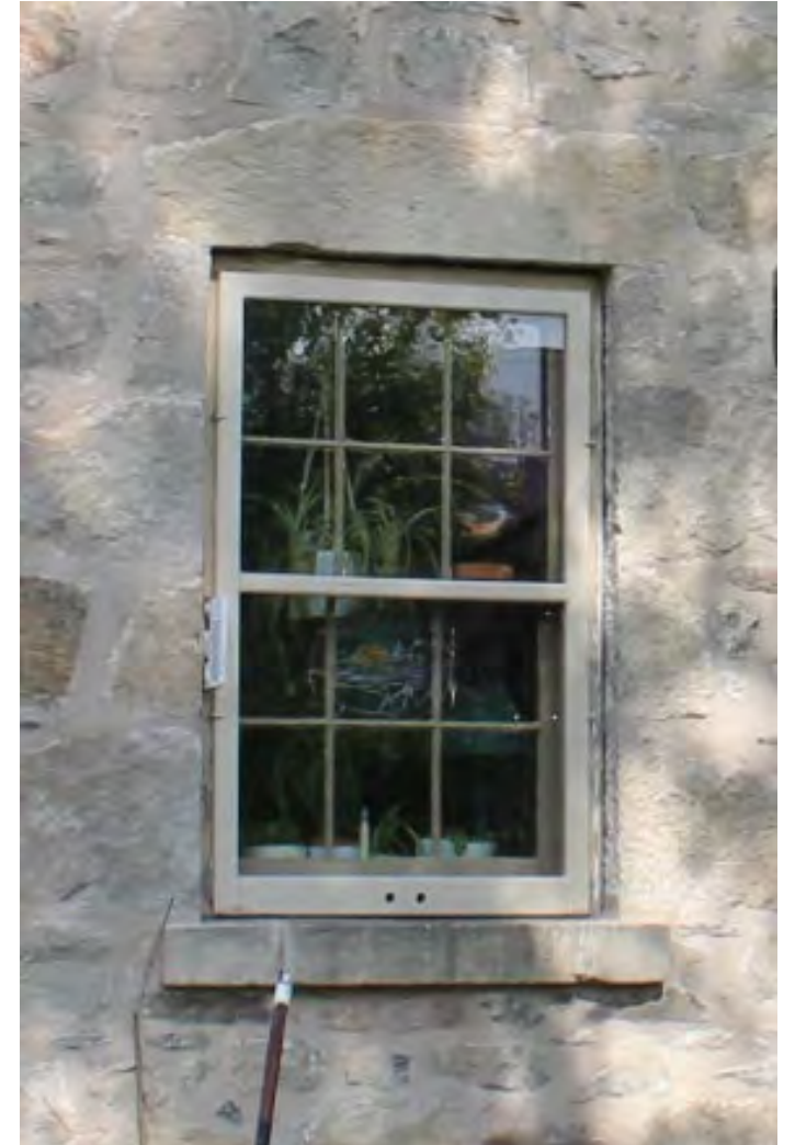
South Elevation Lower Window
