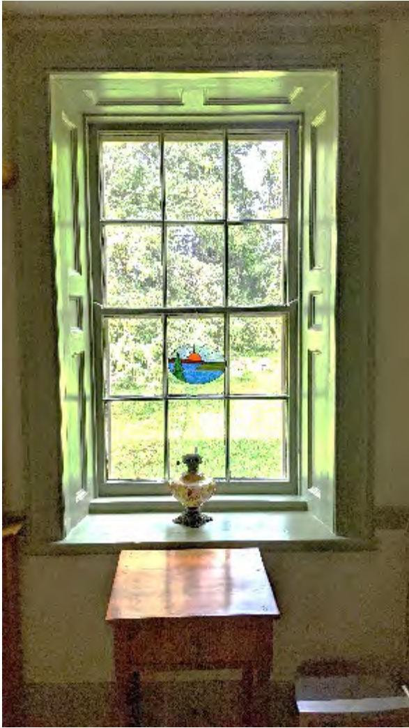
Interior View of Windows
