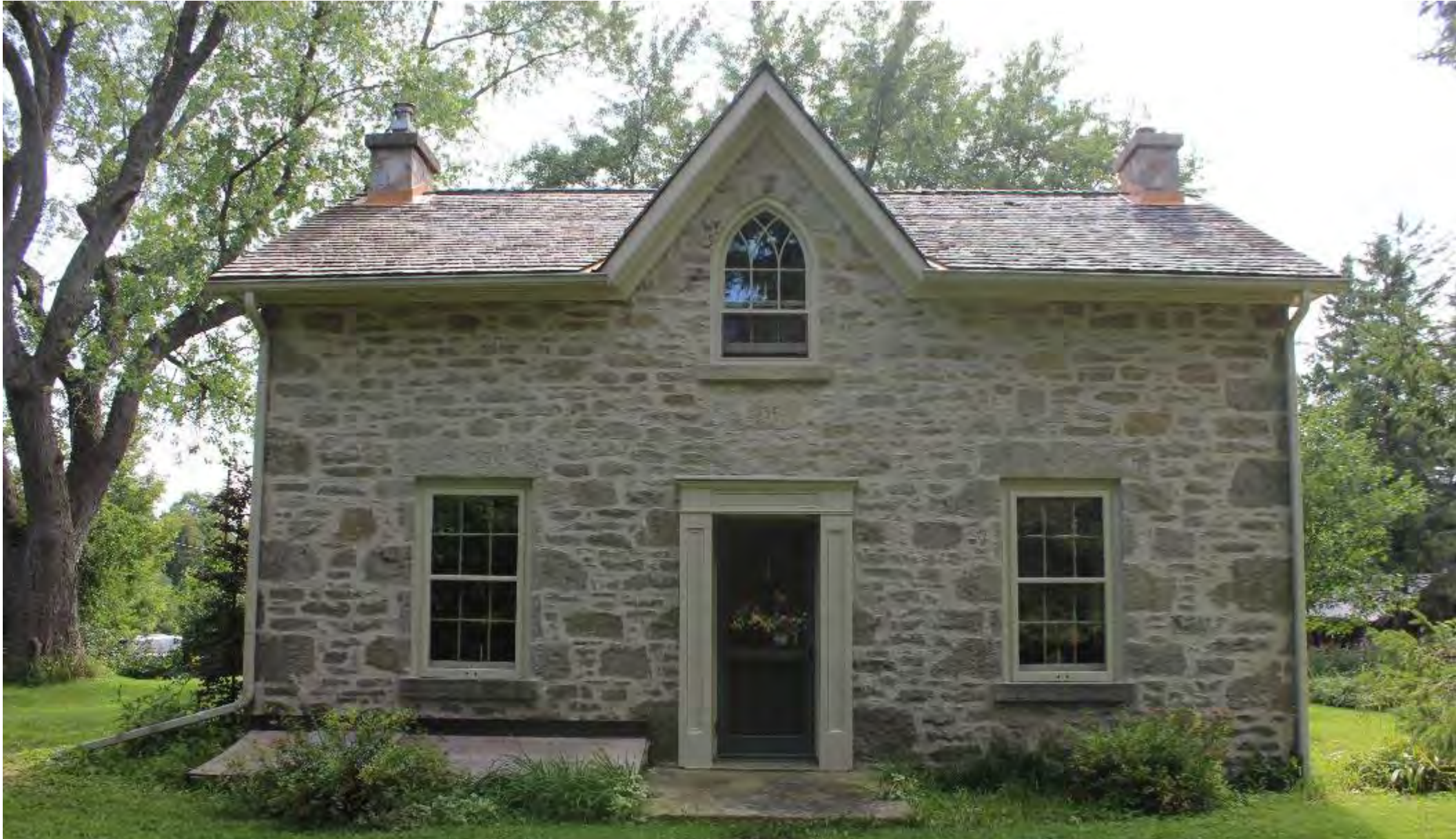
North Elevation _ Cedar Roof Replacement, Cross Gable and Gothic Window added 1984
