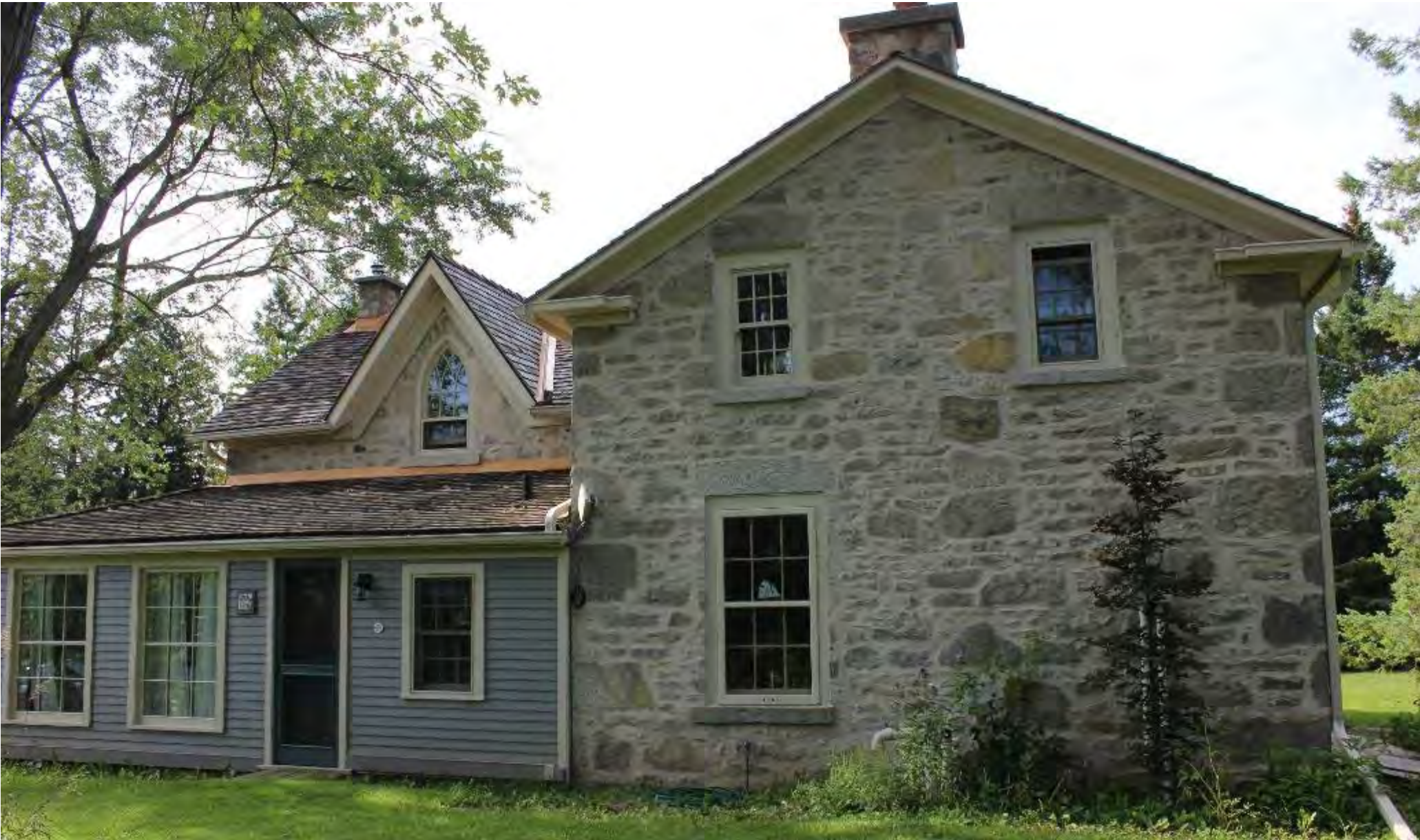
East Elevation_ Cedar Roof reinstallation, Cross Gable and Gothic window added 2014
