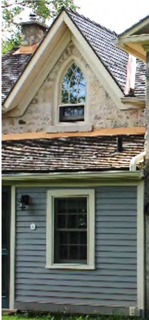
East Elevation Gothic and Six over Six Windows
