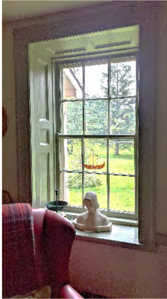
Interior View of Windows
