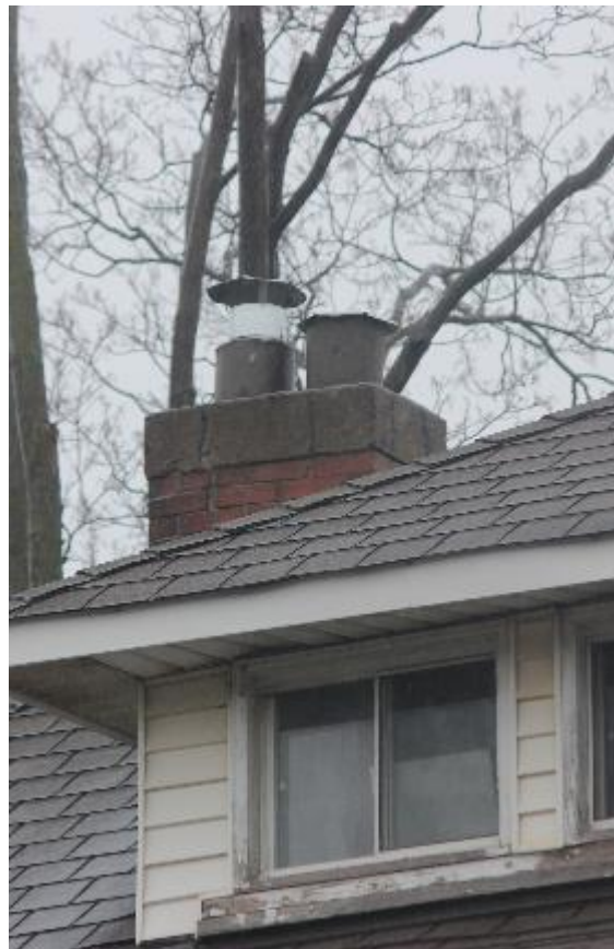
View from North
