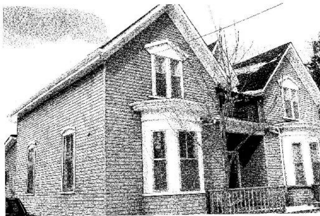
Built in the Victorian Gothic style this home has twin gables facing the street with one-storey bay windows and double unit, pediment topped windows above. The recessed entrance has a gable above.
