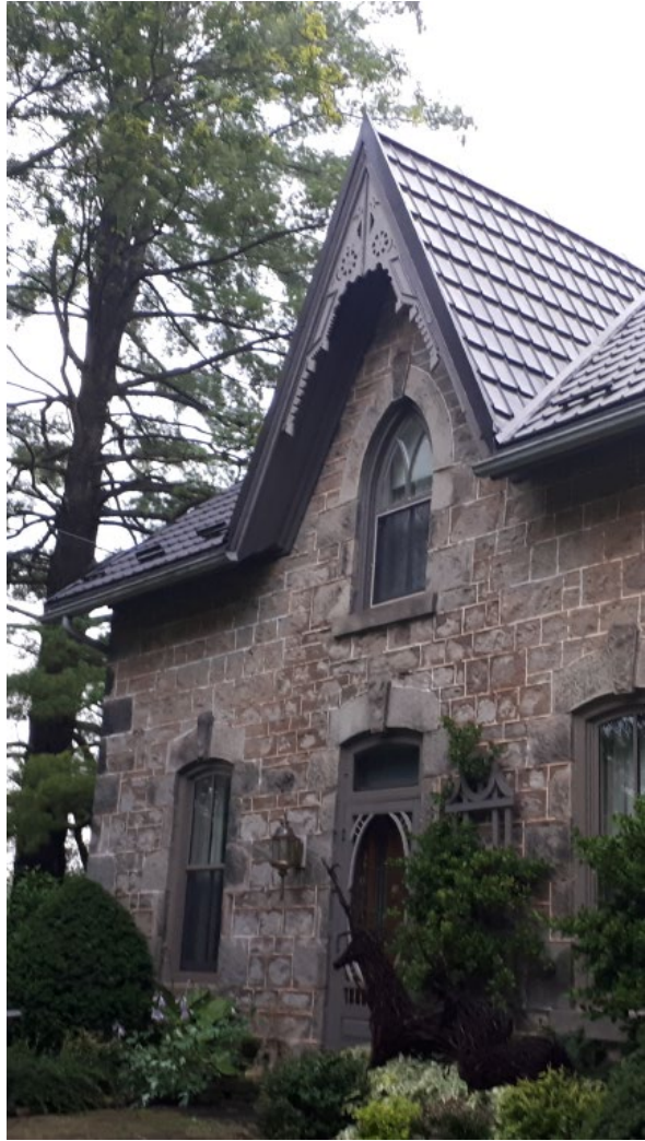
Decorative Verges on the North Elevation
