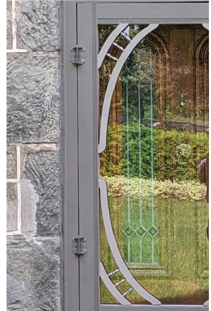
Stain Glass Insert Detail
