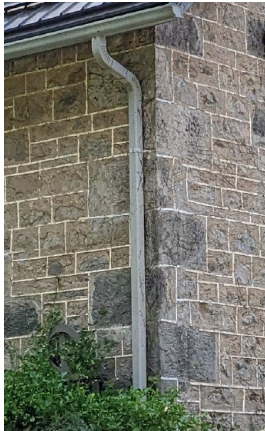
North West Corner
