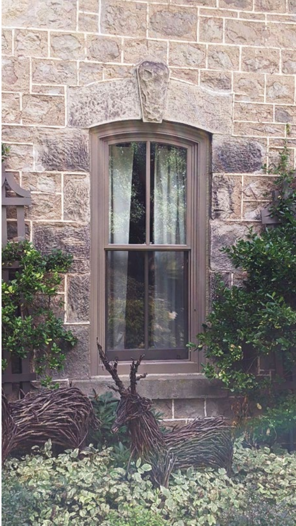
Ground Floor Window North elevation
