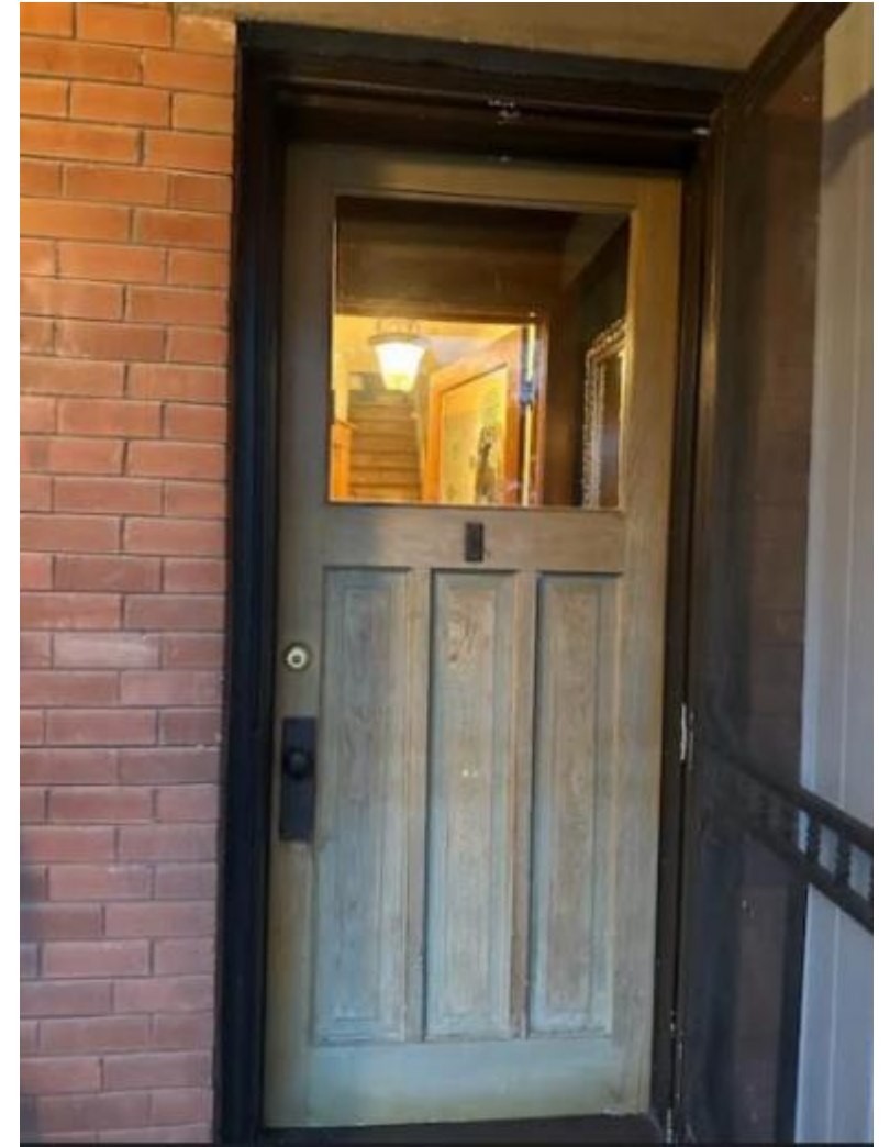
View from Exterior
