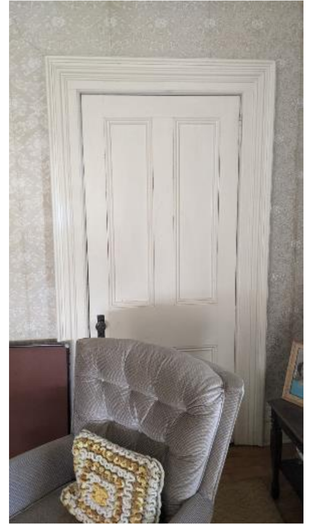
Interior Door with trims
