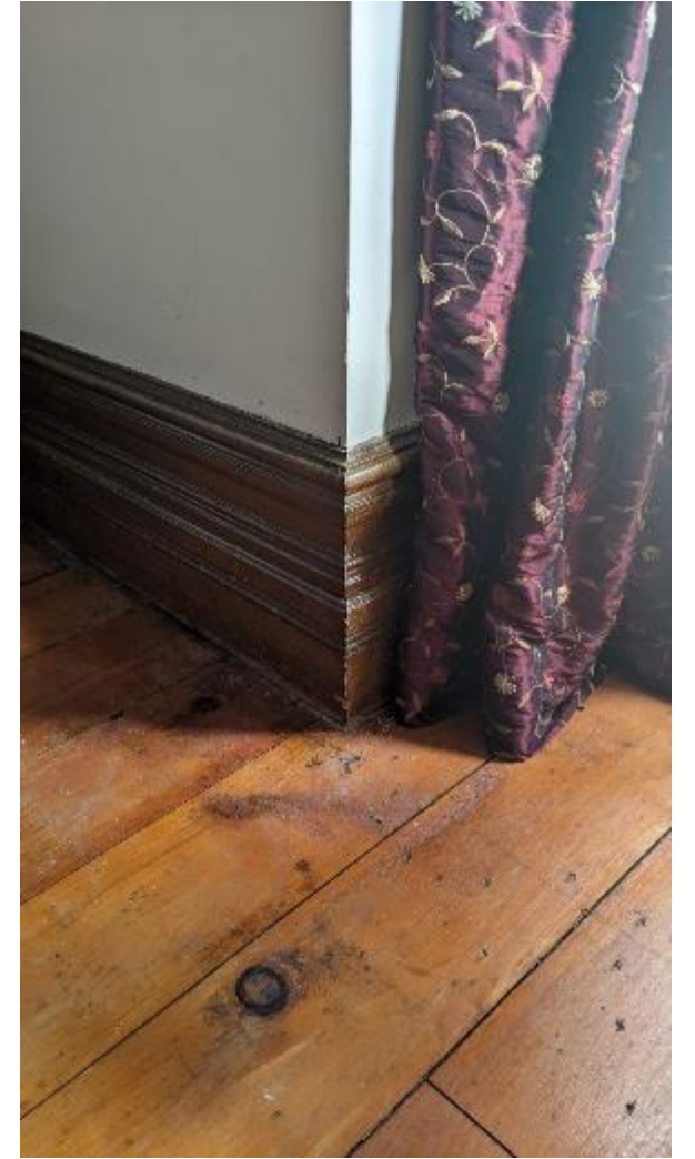
Original baseboard trims
