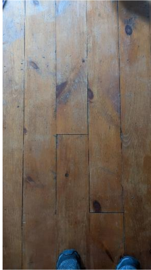
Original wood flooring
